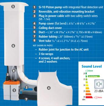
Plug in power cable with two safety switch wires Pump cover (flat bend) L 6<sup>1</sup>/<sub>2</sub>" x W 6<sup>1</sup>/<sub>2</sub>" x H 2<sup>3</sup>/<sub>8</sub>" 6 Duct − L 30" x W 35/32" x H 23/8" (L 750 x W 80 x H 60mm) **7** Rubber tubing L 20" (500mm) x 19/32" i.d. (15mm) 8 Vent tube 5/32" i.d. x L 2 15/16" (4 i.d. x L 75mm) Rubber joint for junction to the AC unit
